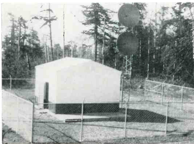
Fig. 2: Typical remote repeater station. Cost of transmitting and receiving equipment is only small part of total cost.
