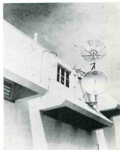
Fig. 3: Simple pipe-mounted installation
